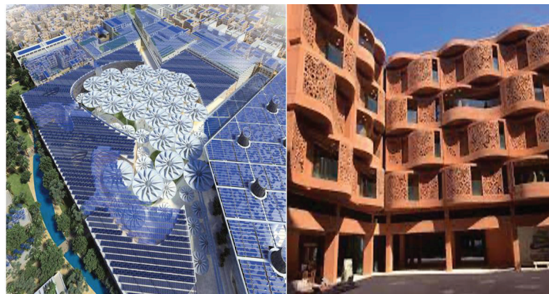
Figure 3: The Masdar City, United Arab Emirates, a Sustainable Mixed-Use Contemporaneous eco-city Model. Photos, Foster and Partners web.page.
