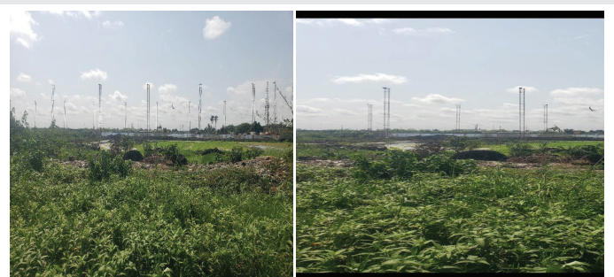
Figure 4: Coastal area dredging, leading to clogged water and vegetation destruction.
